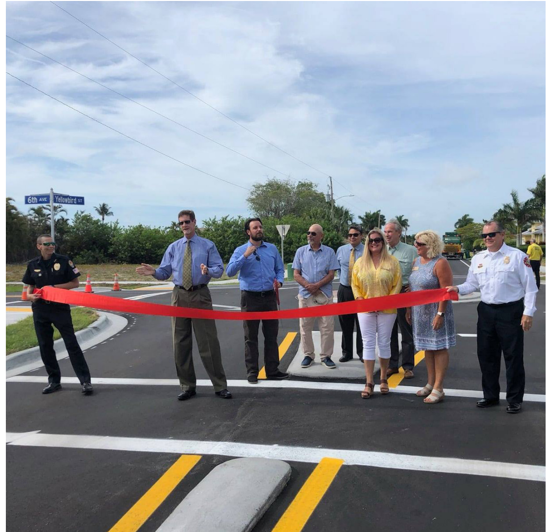
Above: Local partners celebrate completion of work on Marco Island's Yellowbird Road.
